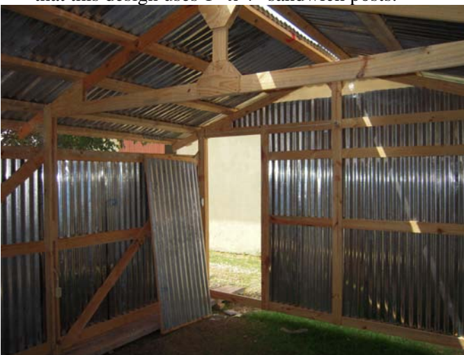
11. View from the interior of the 15m 2 shelter.
