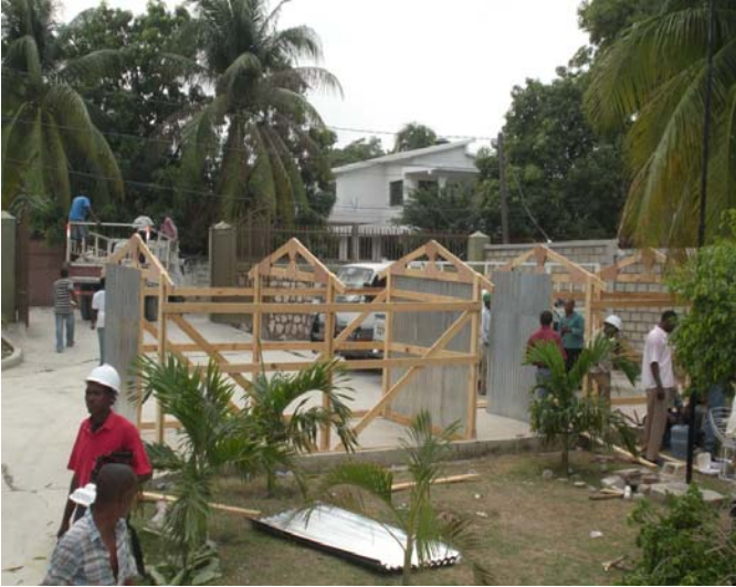
7. Transitional shelters being assembled at the relief center at Delmas 19, Port-au-Prince.
