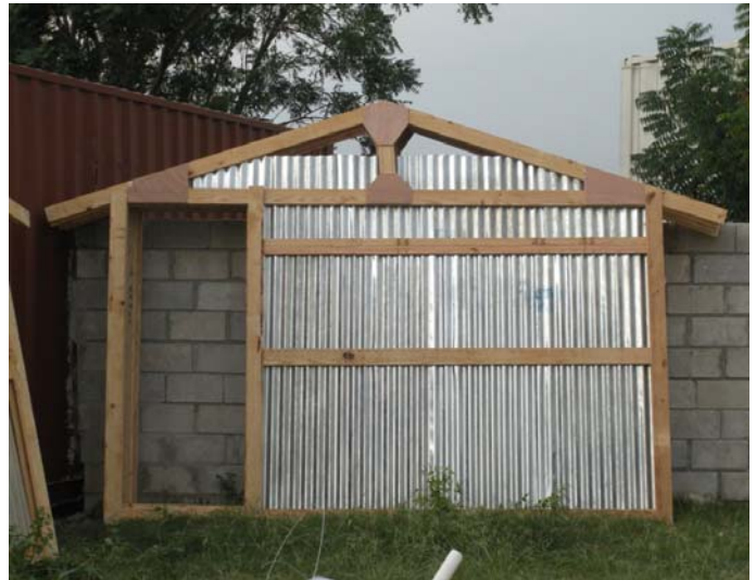
4. Completed end panels with door opening.
