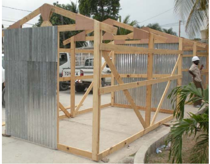
8. Close up of timber structure for the 10m 2 shelter.
