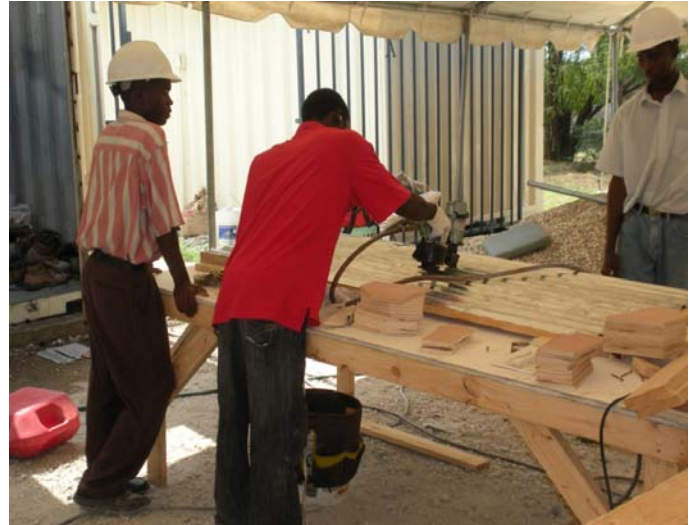
2. Corrugated galvanized iron being applied to the wood frame doors.
