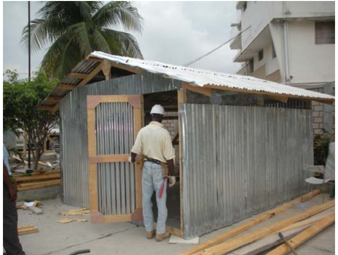
10. A 15m 2 shelter that measures 12' x 14' being built.
