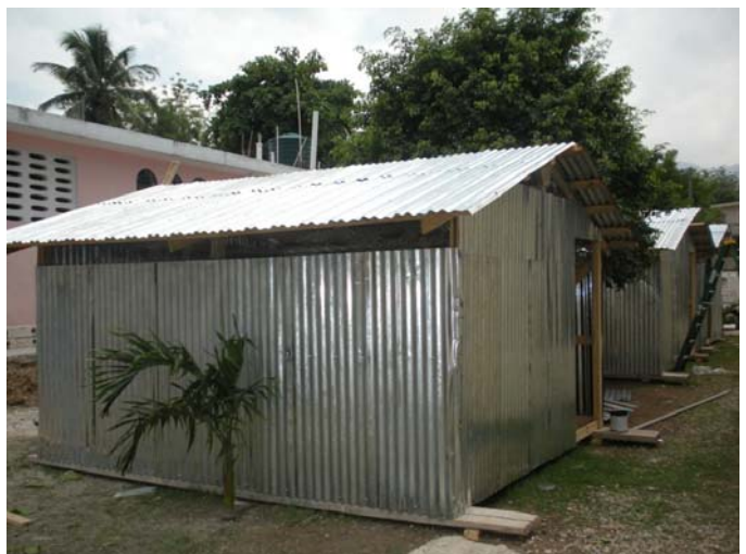
12. Three completed 15m 2 shelters.
