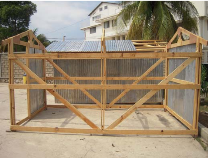
9. Side view of structure for the 10m 2 shelter. Notice that this design uses 1" x 4" sandwich posts.
